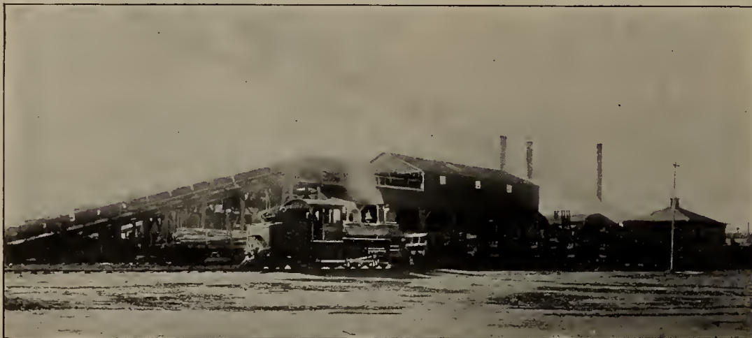
COLLIERIES AT WESTVILLE, NOVA SCOTIA.
